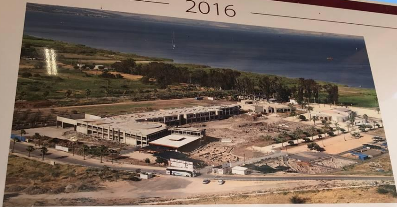
Progress of the construction of the Guesthouse
