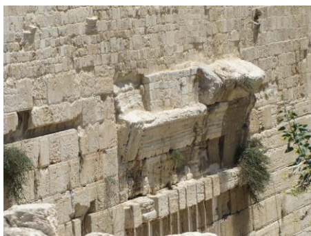
The supporting spring stone that connected the arch to the wall.
