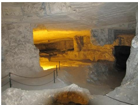
The stone ashlars were taken from this quarry. The straight cuts and grooves of the square blocks that were removed can still be seen.
