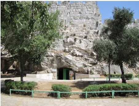
The entrance to Solomon's Quarries (or, Zedekiah's Cave) in the north wall just east of the Damascus Gate.
