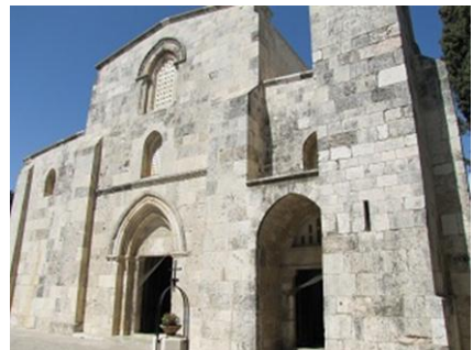
The facade of the Crusader church dedicated to St. Anne. In front of the church is a plant setting on the opening of a cistern to access to water below.
