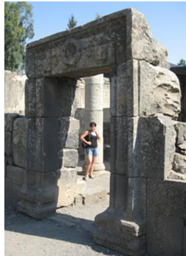
Toni stands inside the north entrance of the synagogue built with ashlars, no mortar and a lintel with a carved wreath.
