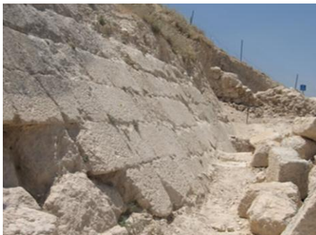
The sides of Herodion were covered with flat stone like armor all the way around from the bottom to the top.
