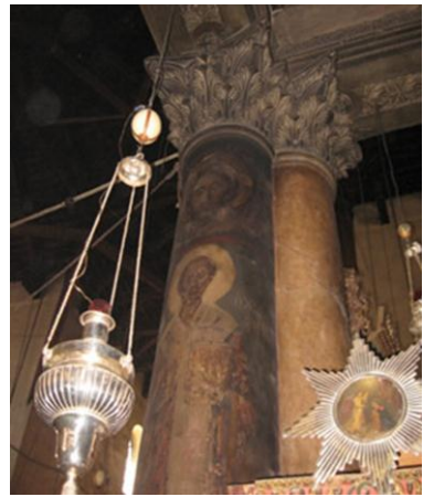
19.5' polished limestone columns of 325 AD with corinthian capitals covered with frescoes (pigment melted into wax) of the Apostles by Crusaders in 1100 AD
